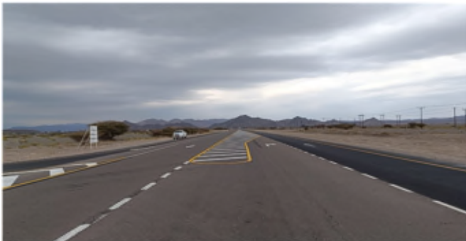
Project junction & signboard (left centre)
