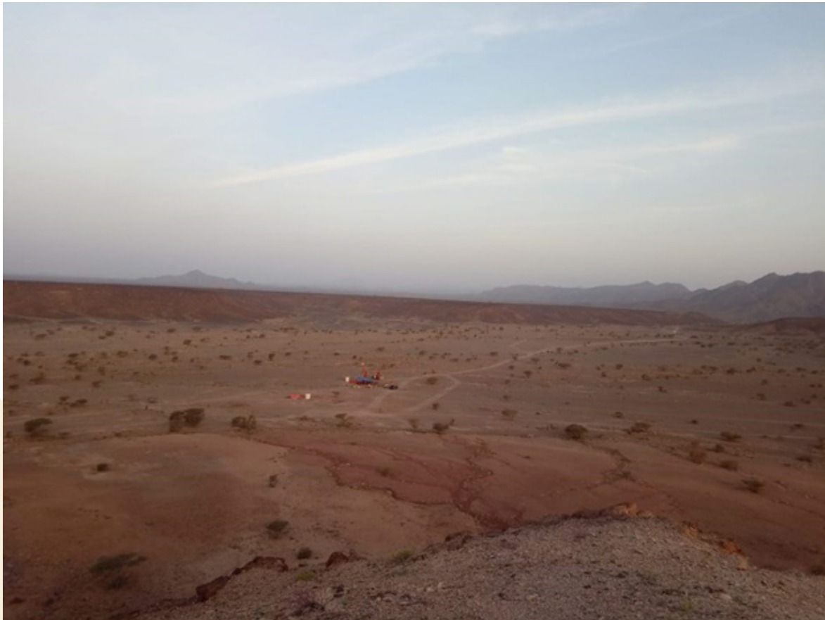
Wash-hi Majaza project site with ARL drilling rig in operation.
