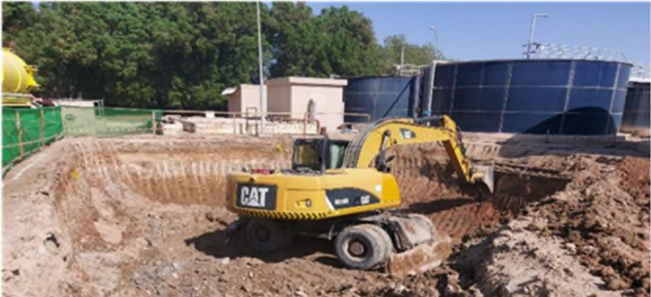
Figure 4: Tank excavation works at the Haya Water site
