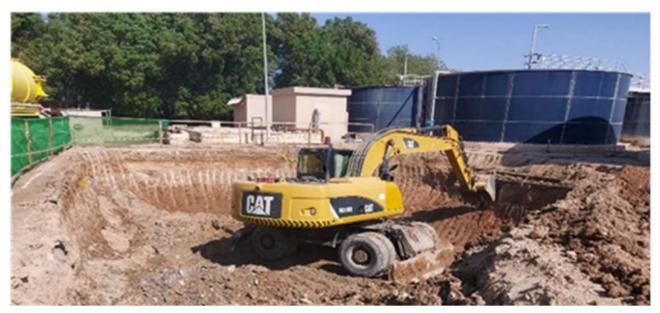
Figure 5: Tank excavation works at the Haya Water site
