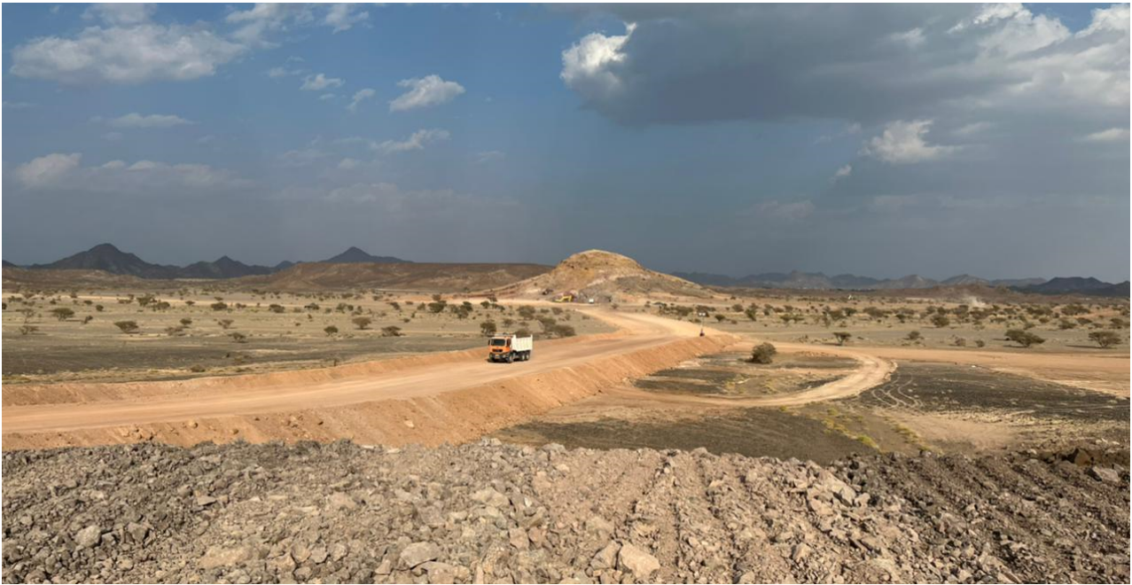
Image 3: Waste haulage road constructed
