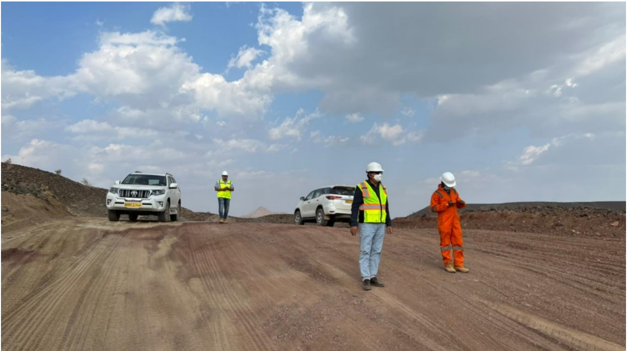
Image 4: Ore haul road under construction
