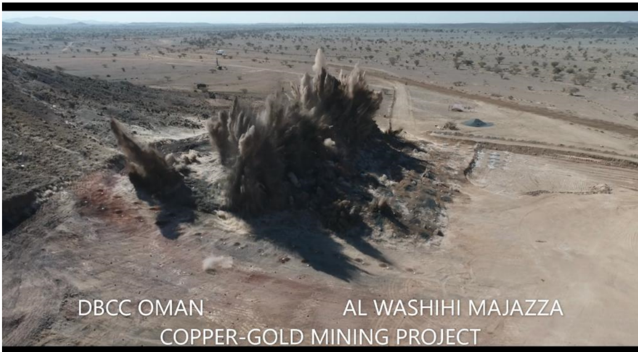
Image 1: First controlled blast at Wash-hi Majaza site
