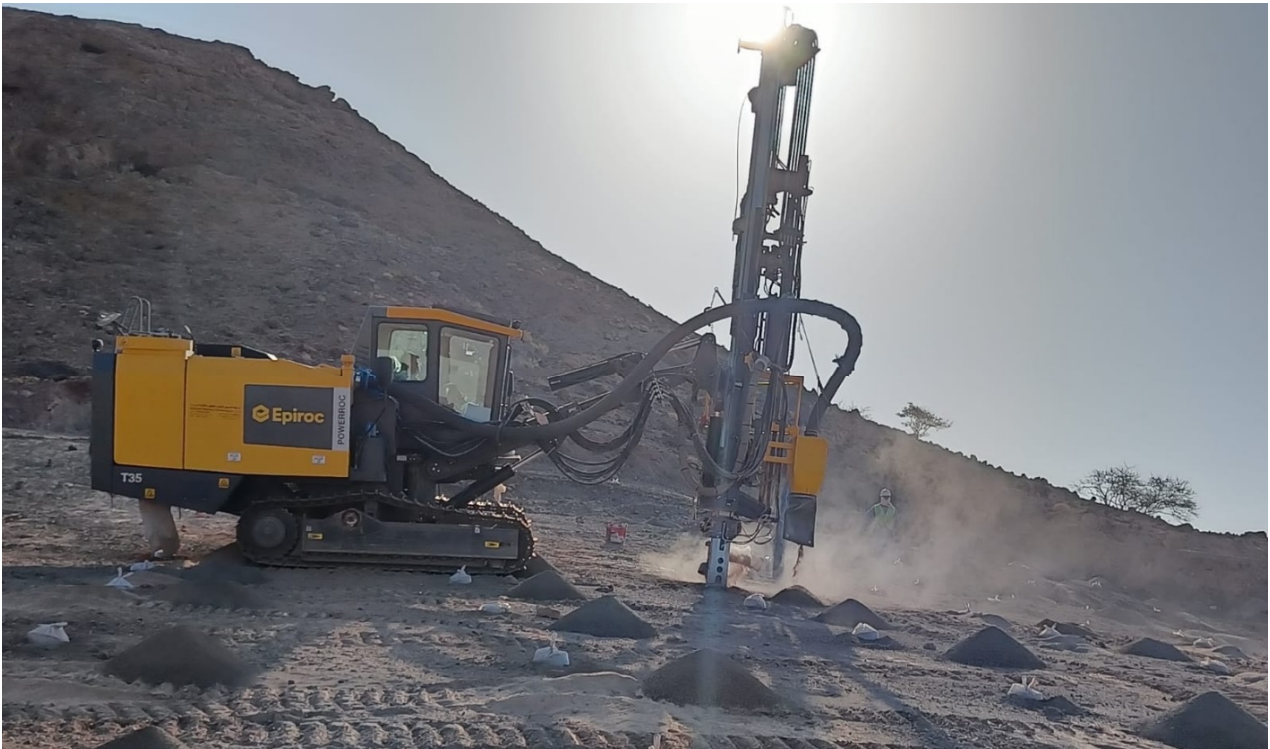
Image 6: Drilling in progress
