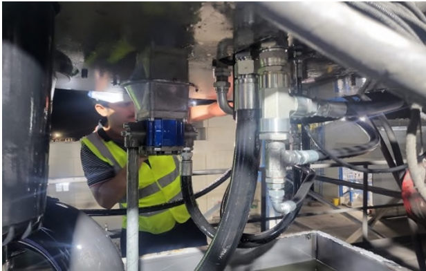
Image 1: Checks on hydraulic unit
