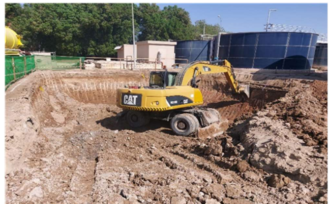
Tank excavation works
