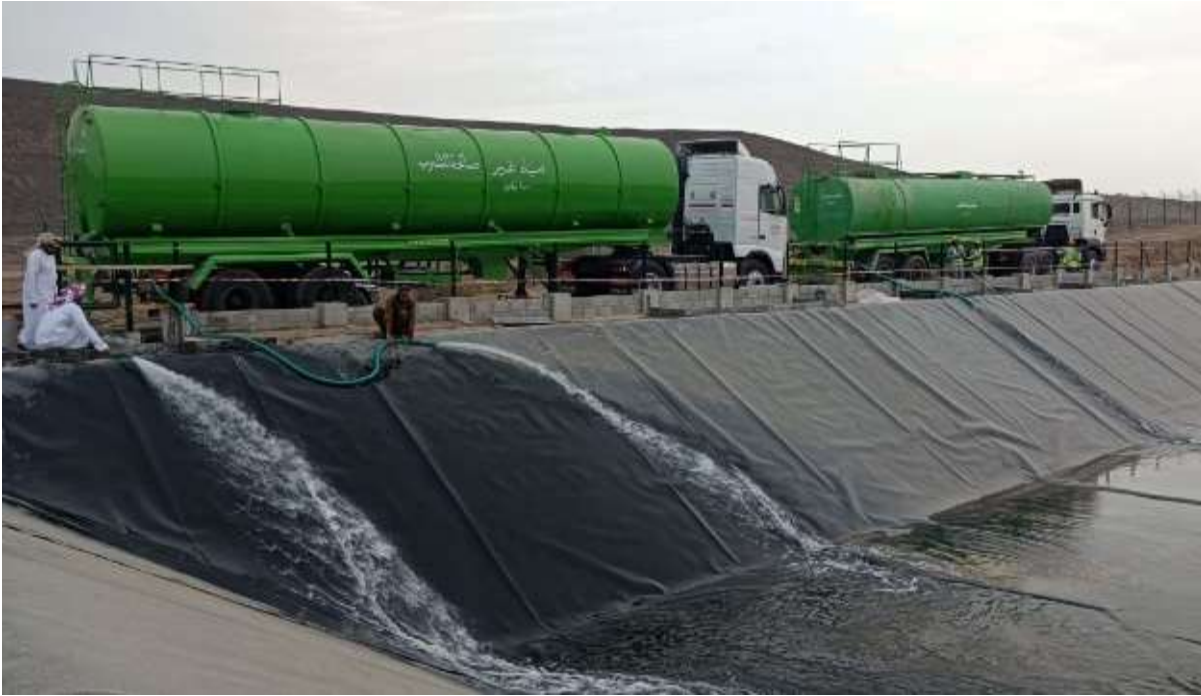
Water storage tank first fill
