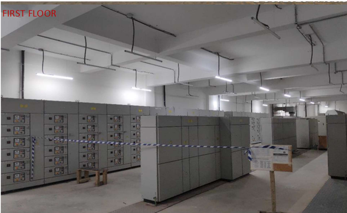
Grinding electrical room – first floor
