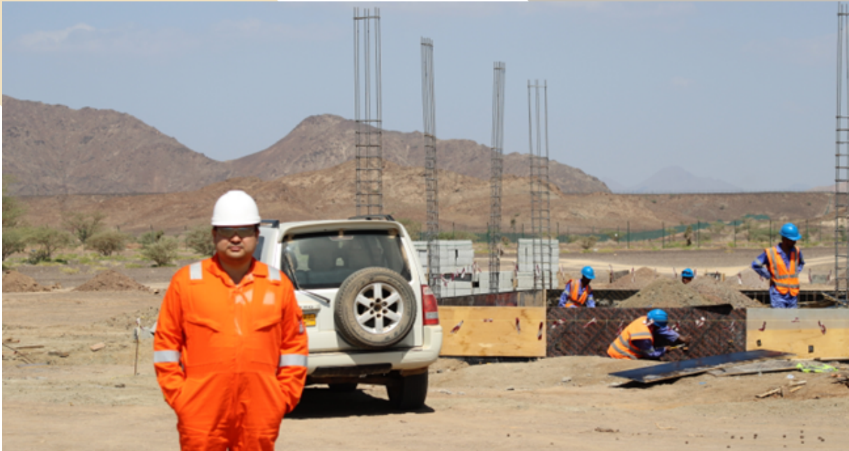
AHRL CEO Avigyan Bera inspecting mining camp foundations
