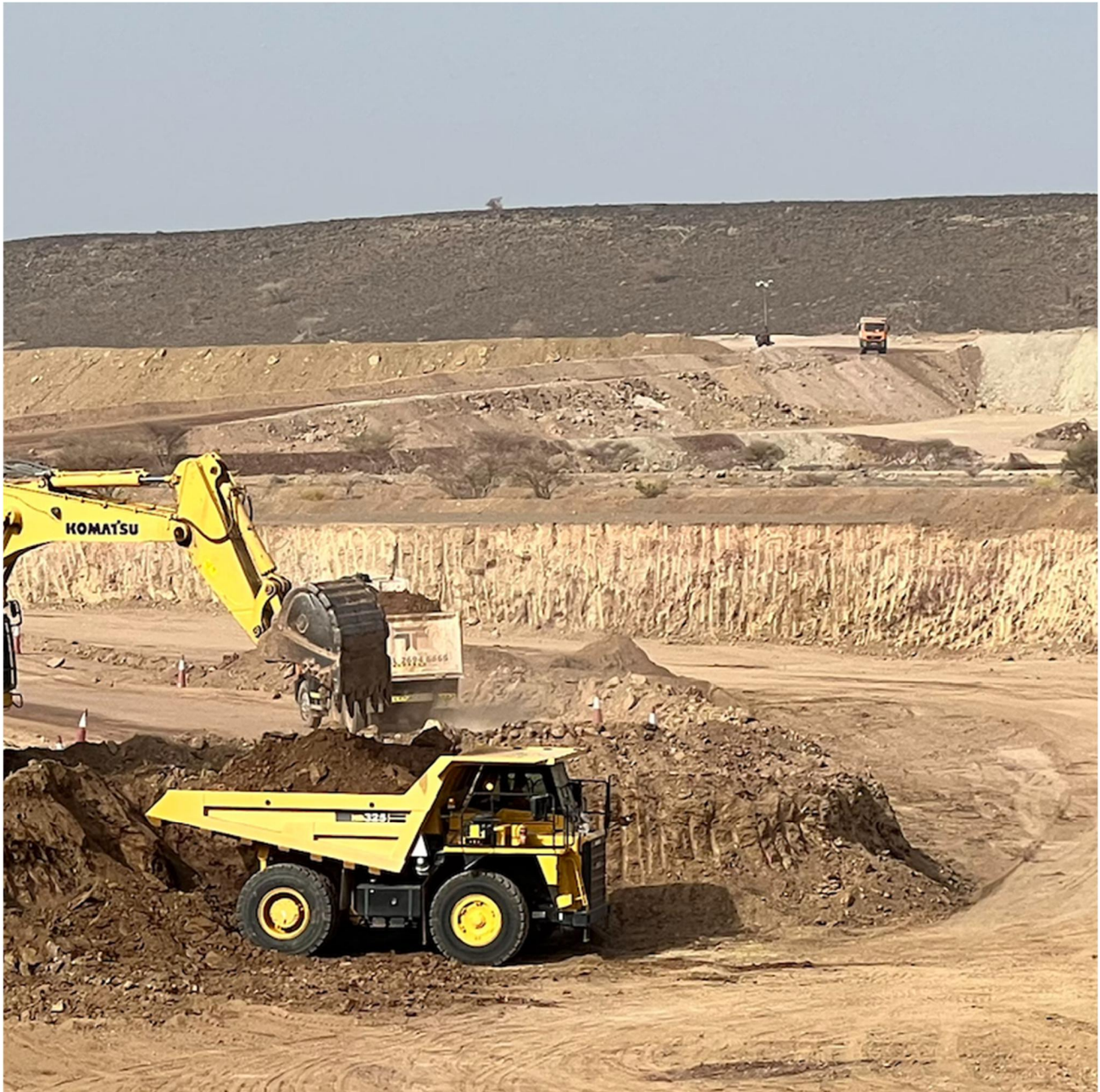
Looking west – Overburden pre-stripping and waste rock area development
