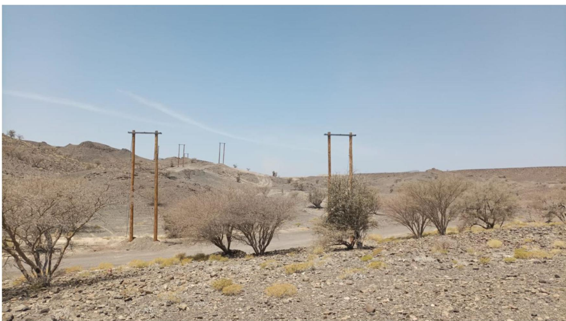
Power feeder poles erected
