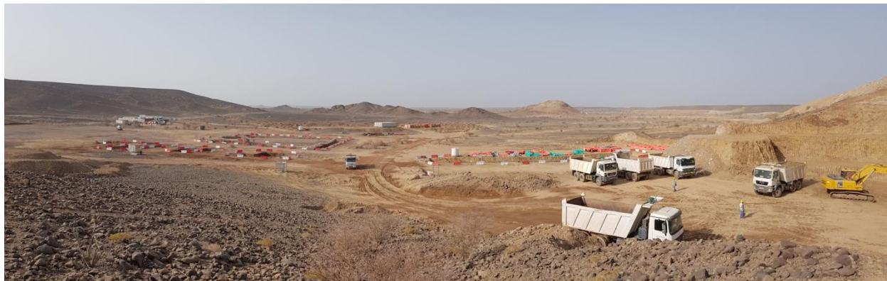
Primary crushing unit and retaining wall site development #1
