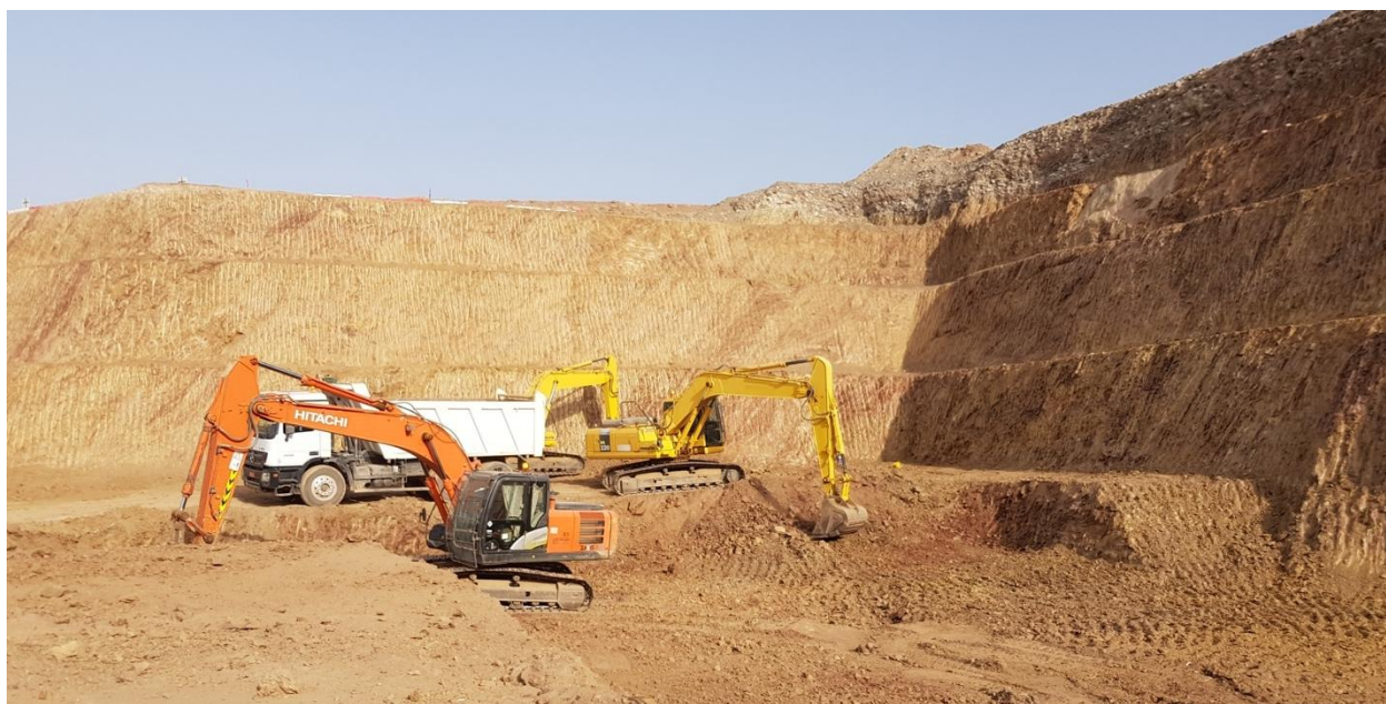
Primary crushing unit and retaining wall site development #2
