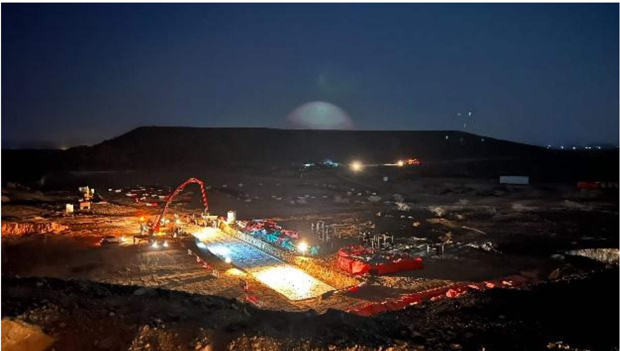
Concrete pouring at crushed ore stockpile and belt conveyors BC – 02 & 03
