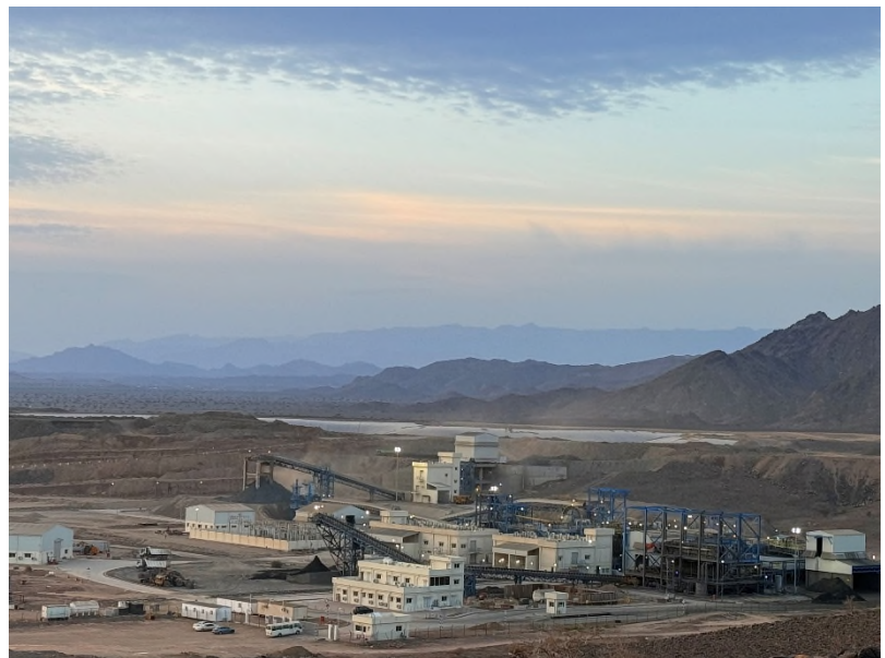
Image: Wash-hi copper-gold processing plant
