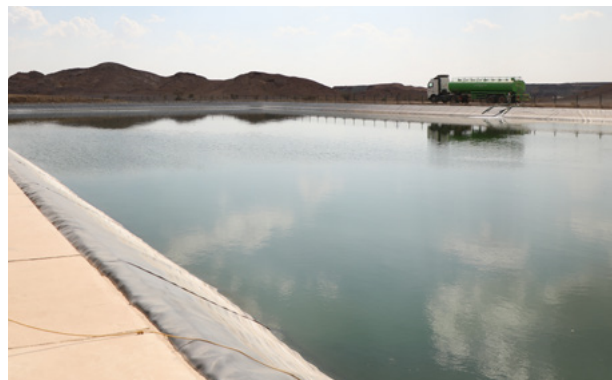
Fresh water storage facility
